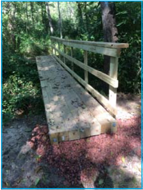
New bridge on Buckeye Trail at Tappan Lake Park
