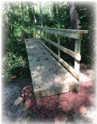
New bridge on Buckeye Trail at Tappan Lake Park.
